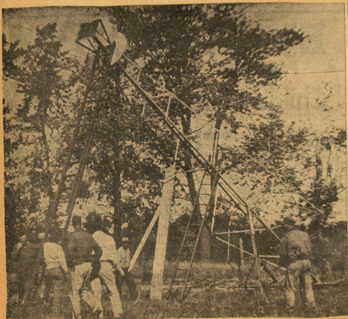
NEW FIRE TOWER — Delafield firemen recently raised a windmill tower for a new fire siren which will double as an alarm for civil defense. In the top picture, firemen put their skill with ladders to work in raising the 40 foot tower. Included in the picture, left to right, are Jim Tietz, Elmer Zellner, August Steinhart, Edward Jaroch, Chief Hugh Roberts and William Roberts.
